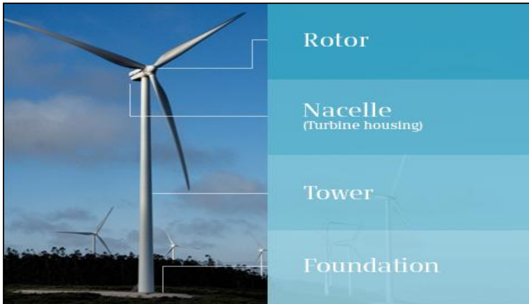
Plate 3-1 Wind Turbine Components
