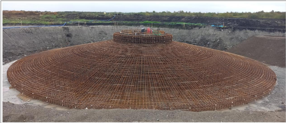
Plate 2-3 Turbine Base Anchor Cage
