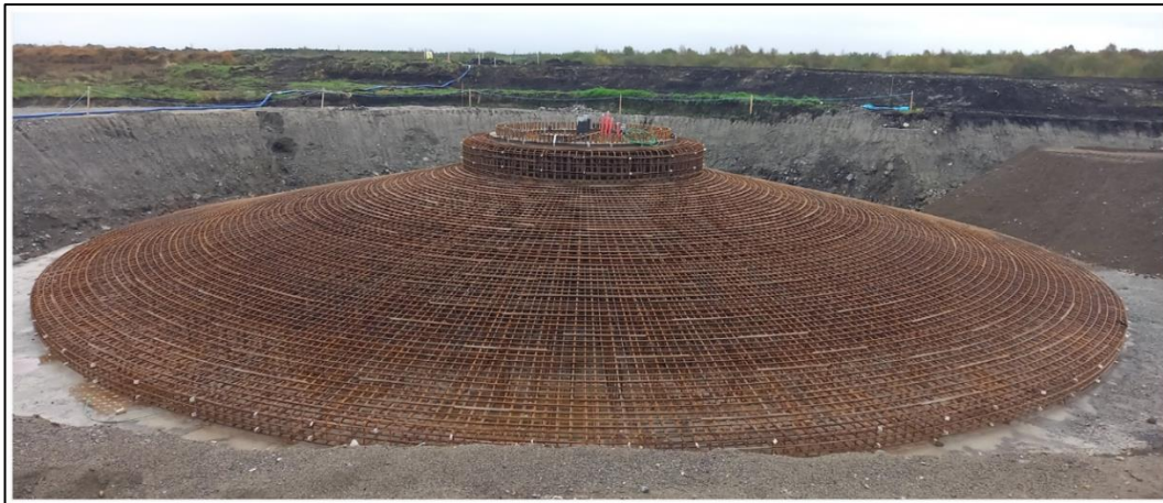
Plate 3-3 Turbine Base Anchor Cage
