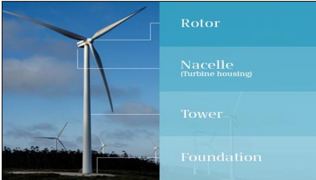
Plate 2-1 Wind Turbine Components
