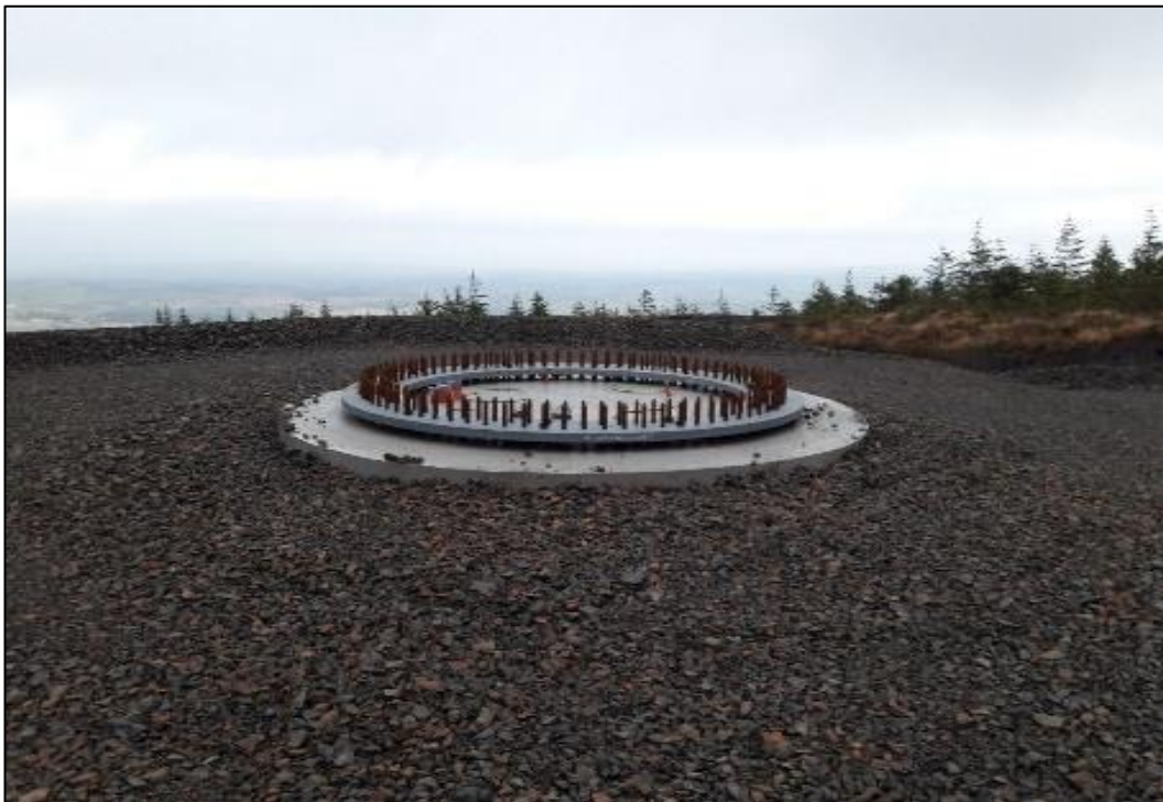
Plate 3-4 Finished Turbine Base
