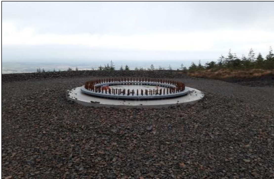
Plate 2-4 Finished Turbine Base
